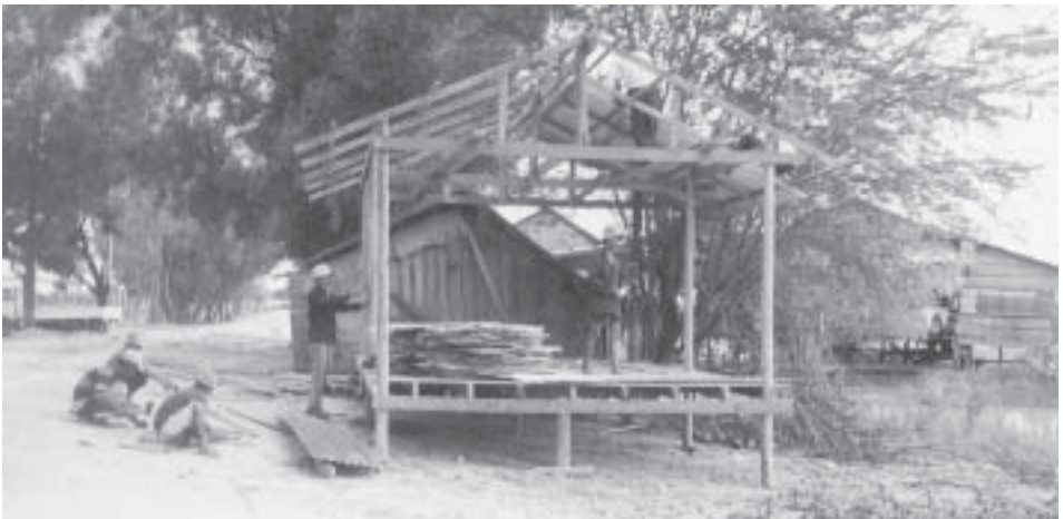
Boeung Chhouk village church under construction. Funds to build this church were given by ASAP donors.
